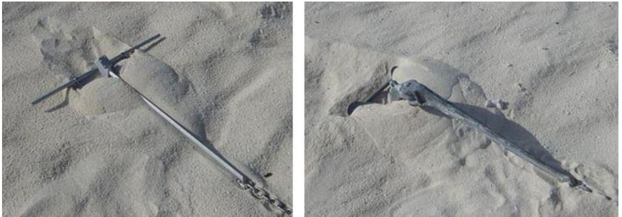
Figure A-6 properly buried anchors
